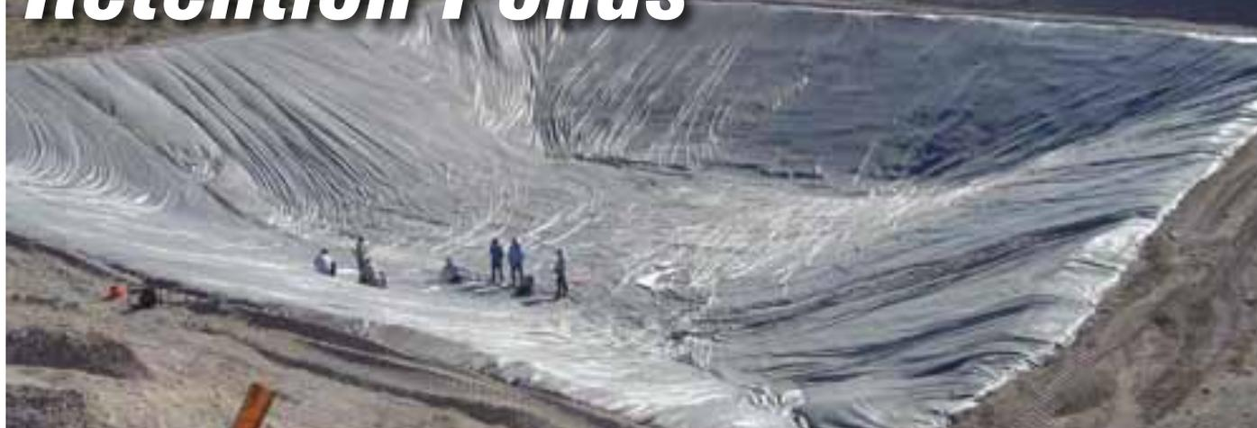
*Ponds can be as small as a backyard water feature or as massive as this oil well waste pit. Either way, the goal is the same: to keep the contents from leaking into the ground.*
