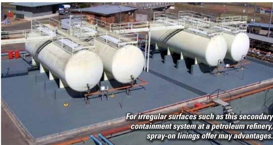
*For irregular surfaces such as this secondary containment system at a petroleum refinery, spray-on linings offer many advantages.*
