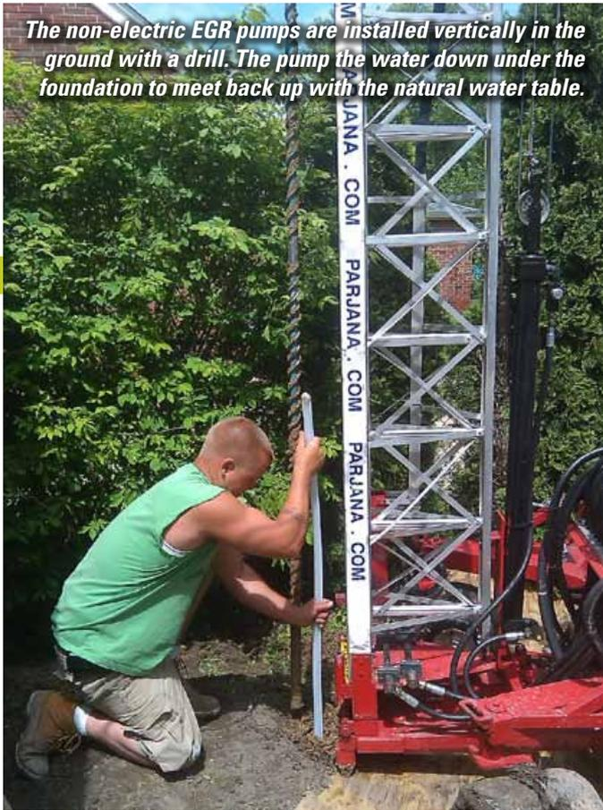
liquid to rise in narrow tubes or to be drawn into small openings such as those between grains of a rock. Capillary action, also known as capillarity, is a result of the intermolecular attraction within the liquid and solid materials. The EGR pump uses the concept of capillary action to bring the water in.
