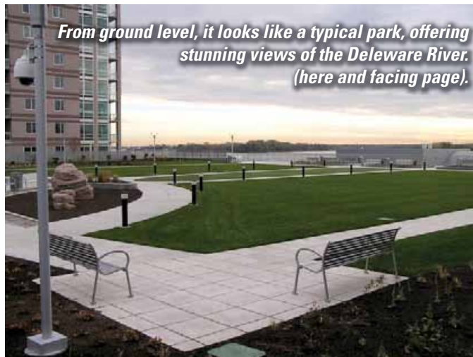
Waterfront Square in Philadelphia used a green deck to improve views from the nearby condo units, provide green space, and mask an underground parking garage .
