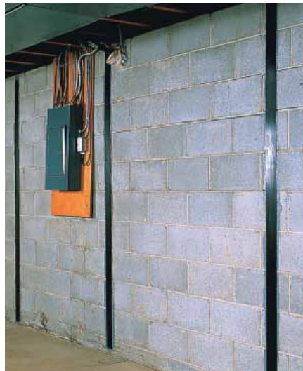
Photo Courtesy of Nationwide Reinforcing
