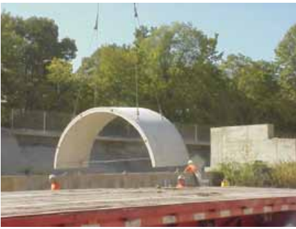
The St. Louis Metro-Link used a bentonite membrane on walls and a butyl rubber on precast roof sections (left and center). Entire pre-cast tunnels like this one in Stamford, Conn. (right) are becoming increasingly common.
