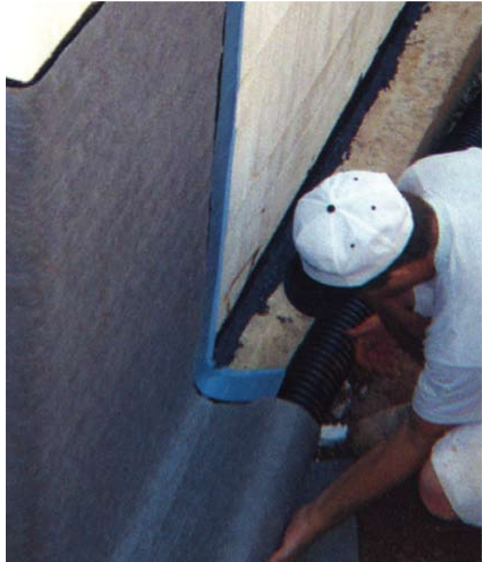
A complete waterproofing system combines an ICF-friendly waterproofing membrane with a sheet drain and drainage tile.
