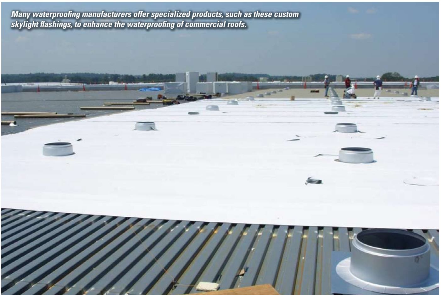
Photo Courtesy Carlisle Syntech
