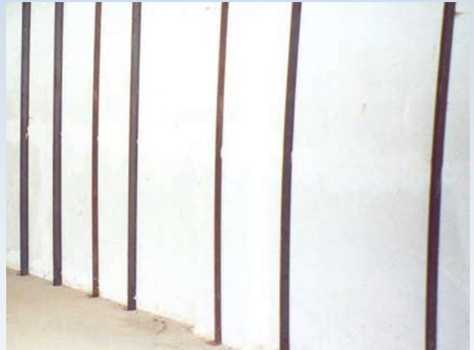
Steel I-Beams, set every four to five feet along the wall, are the traditional solution to fixing bowing.
