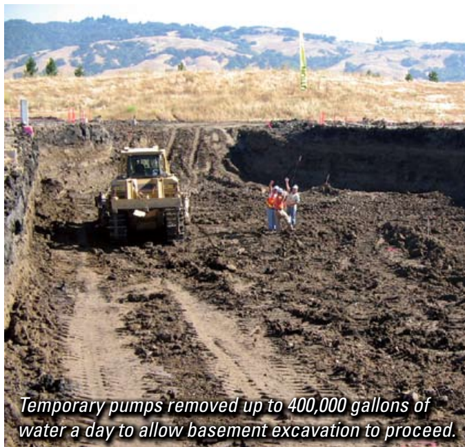
When the dewatering system was shut down overnight, the water table returned to its normal level, 5 feet below grade.
