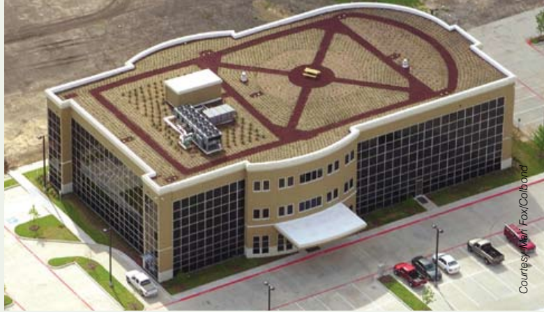
These before and after photos show the installation of a 14,500 sq. ft green roof near Houston. Installed cost was between $10-$15 a sq. ft.
